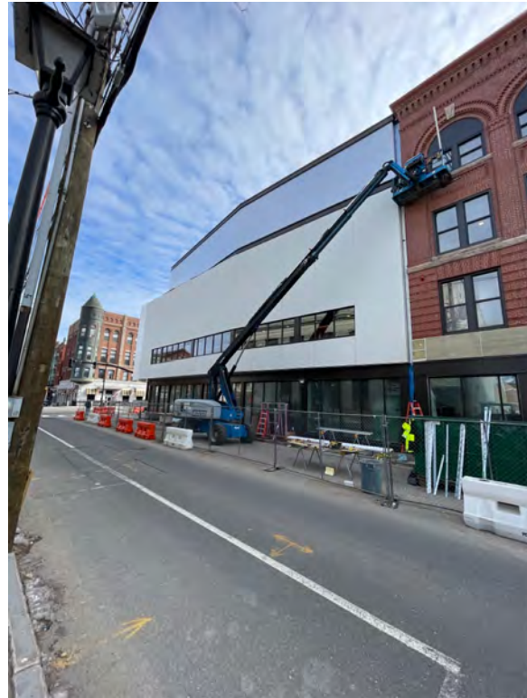
Description: North elevation of addition
