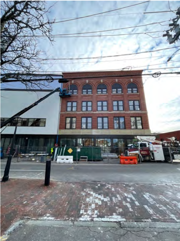
Description: North elevation of existing building
