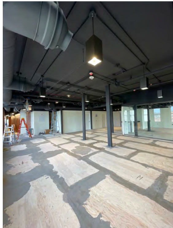
Description: Third-floor existing building
