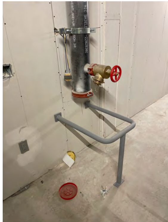
Description: Basement of existing building, miscellaneous metals rails
