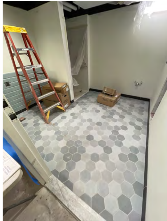
Description: First floor existing tile installed
