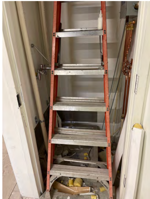
Description: First floor existing, mop sink installed
