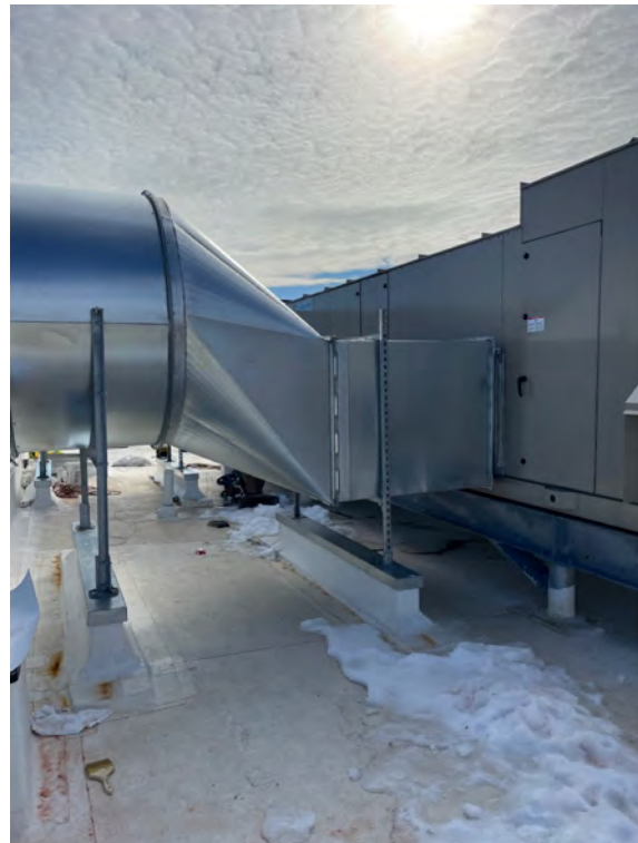
Description: Welding duct terminations
