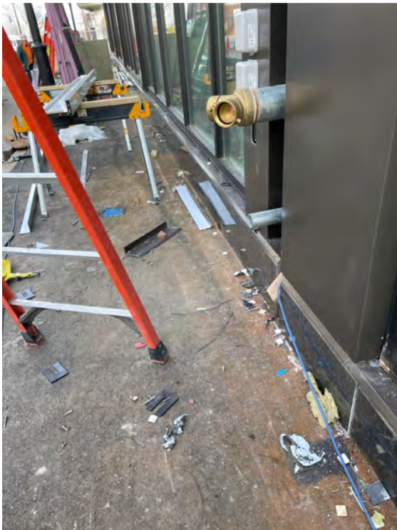
Description: Granite base at north elevation
