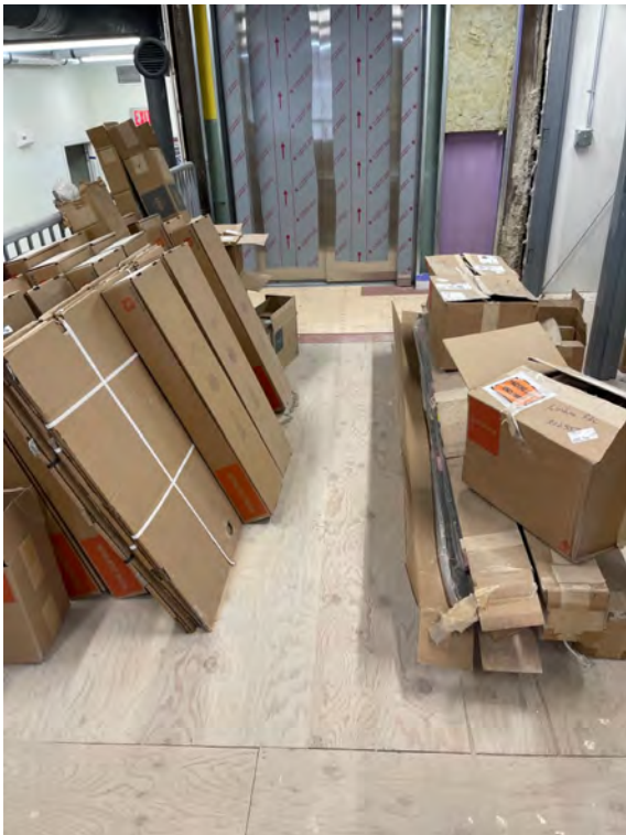
Description: Door hardware on site
