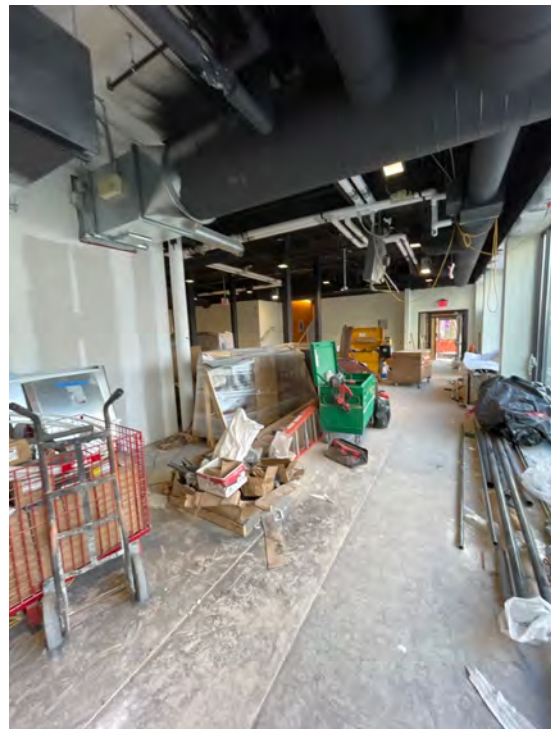
Description: First floor existing building
