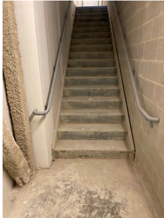
Description: Addition/basement to first floor stairway
