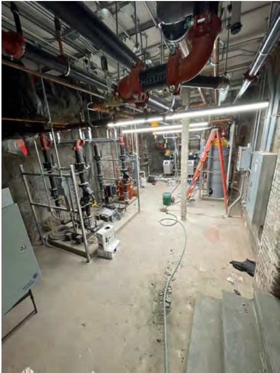
Description: Basement of existing building/Boiler room
