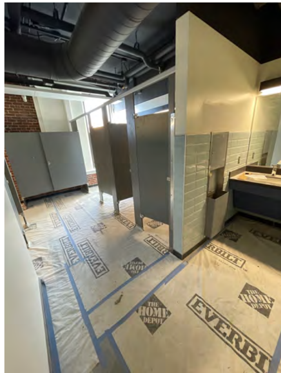
Description: Second floor existing building/gang-bathroom
