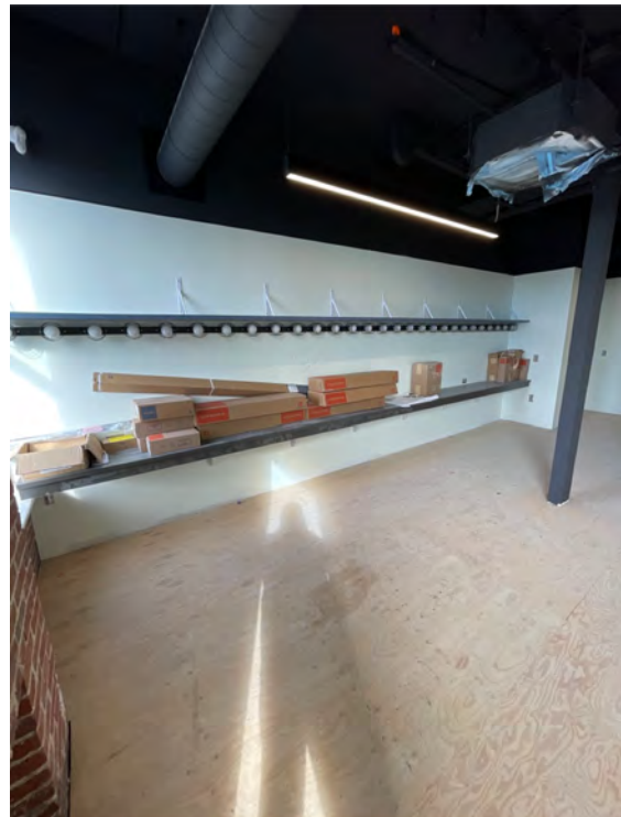
Description: Third-floor existing building dressing room no work and lighting
