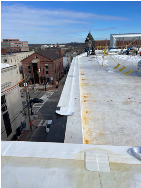
Description: Perimeter metal installation in progress
