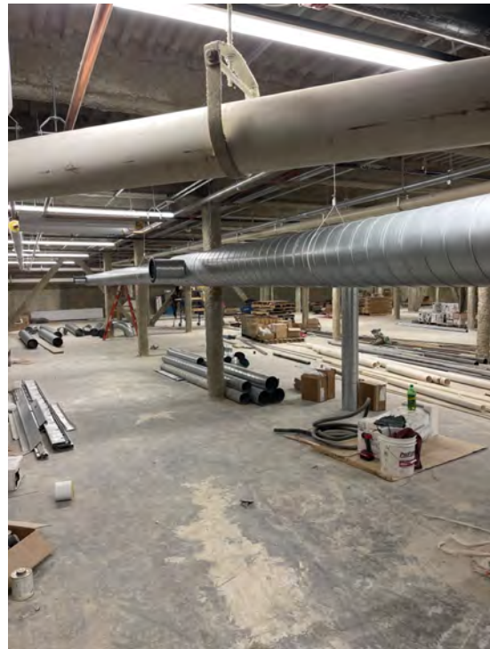
Description: Basement of addition, spiral duct installation in progress
