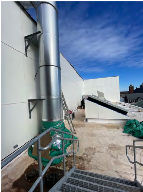
Description: Low roof smoke, hatches, and ductwork installed
