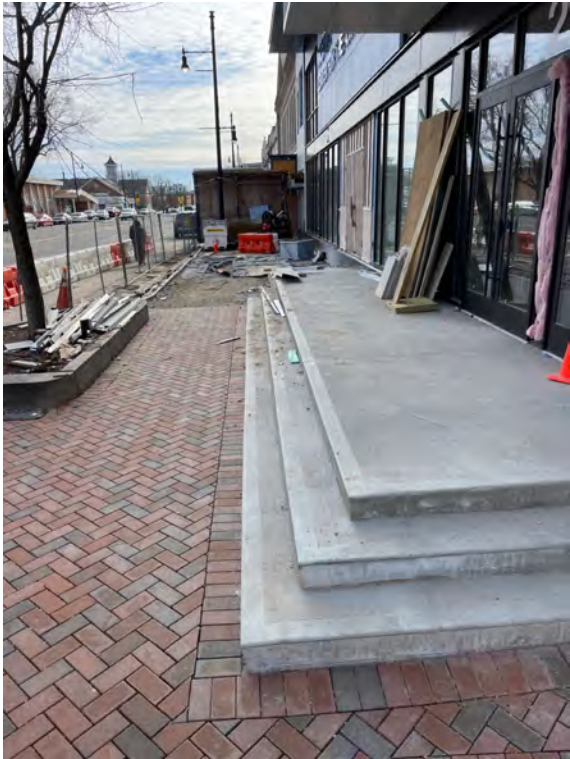
Description: Walkway and concrete installed at East elevation
