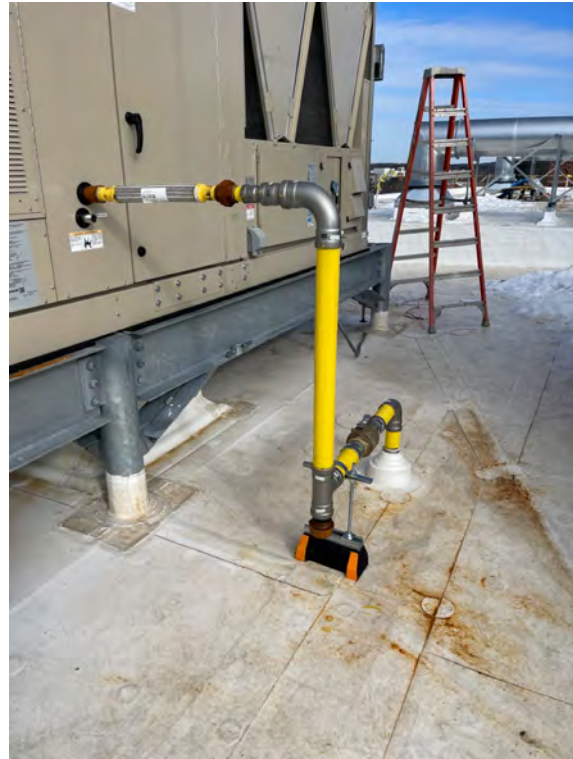
Description: Rooftop unit gas piping final connections, appear complete
