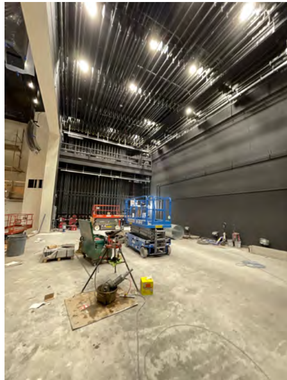
Description: First floor addition stage area/wall priming
