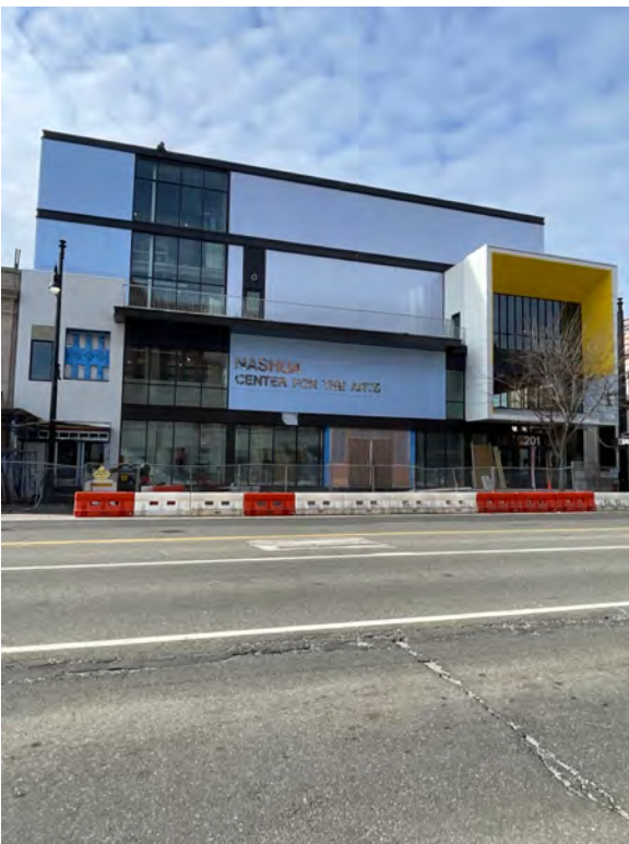
Description: East elevation of addition
