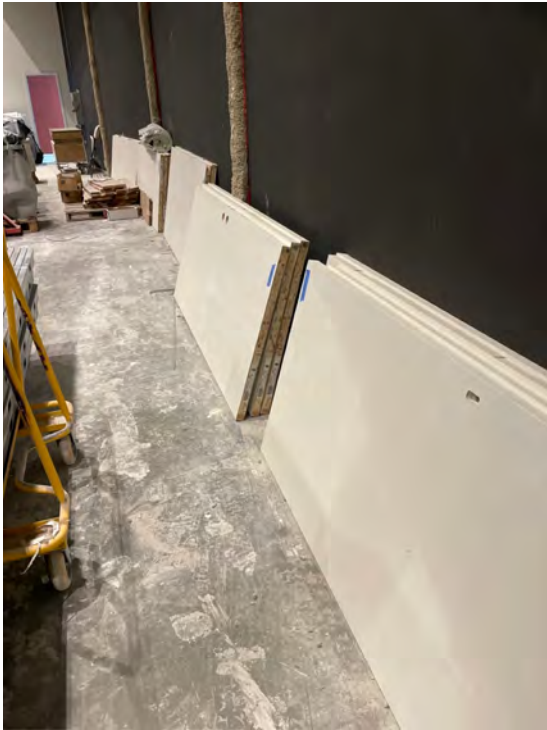
Description: First floor, addition door slabs on site
