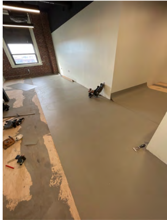
Description: Fourth floor existing building sheet vinyl flooring, installation in progress
