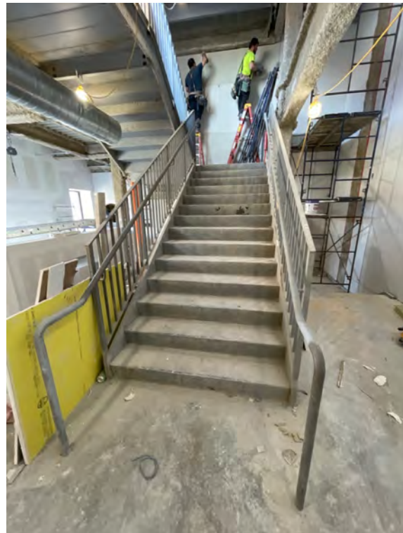
Description: Addition/2nd to 3rd floor stairway
