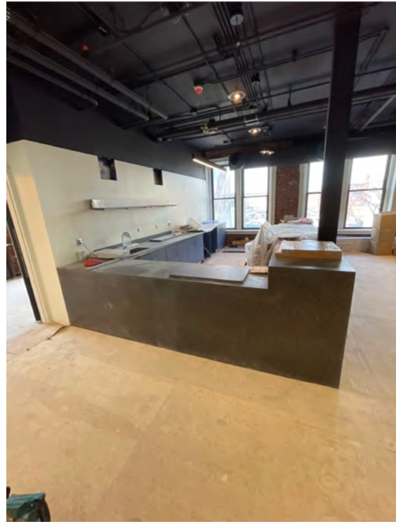
Description: Second floor existing building millwork tops
