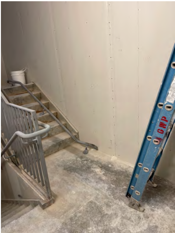
Description: Miscellaneous metals handrails on site
