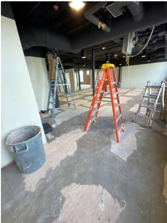
Description: Third floor existing building floor prep in progress
