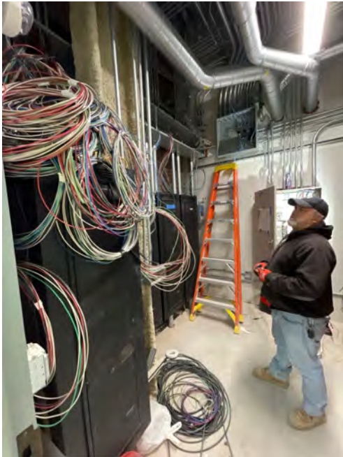
Description: Lighting control room final terminations in progress
