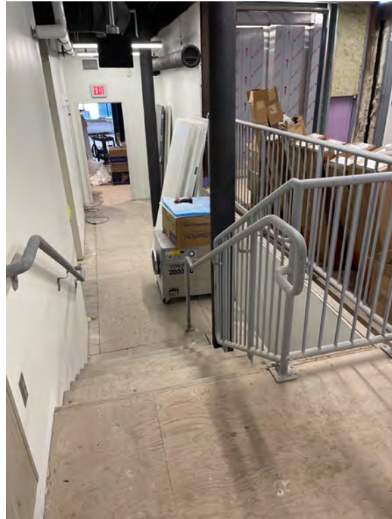
Description: First floor addition/miscellaneous metals, handrails
