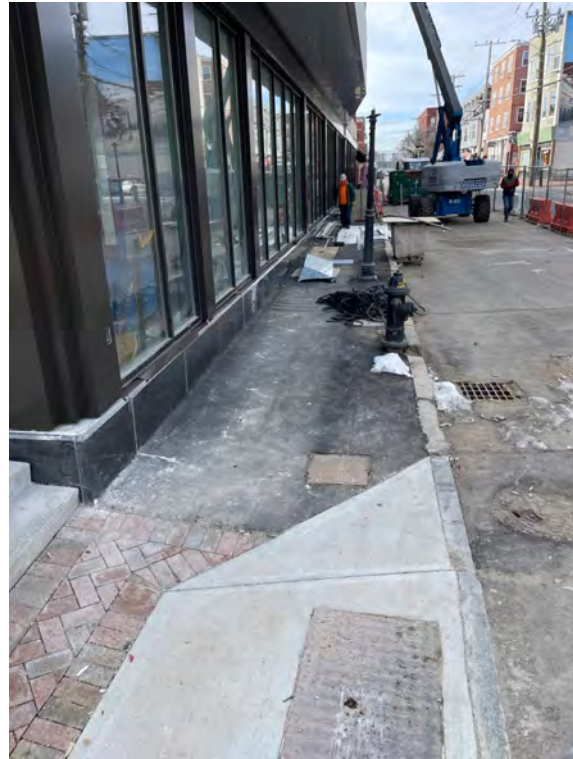
Description: Pavement walkway installed at north elevation
