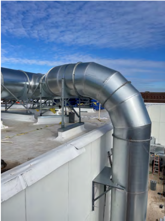
Description: Roof/welded duct installed
