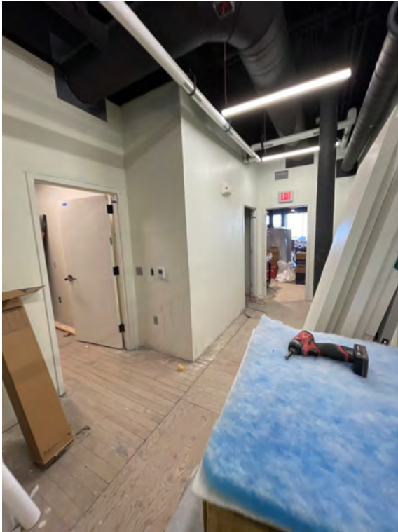
Description: First floor existing building doors, frames and hardware installation
