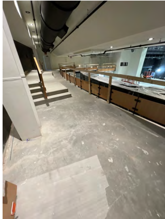
Description: Second floor addition/miscellaneous metals, handrails, and panels
