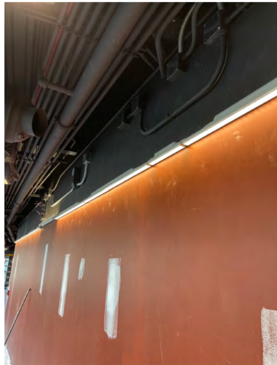
Description: Second floor addition, lighting installed
