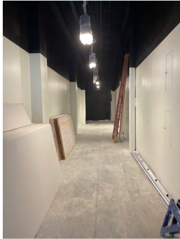
Description: Fourth floor addition/North Corridor
