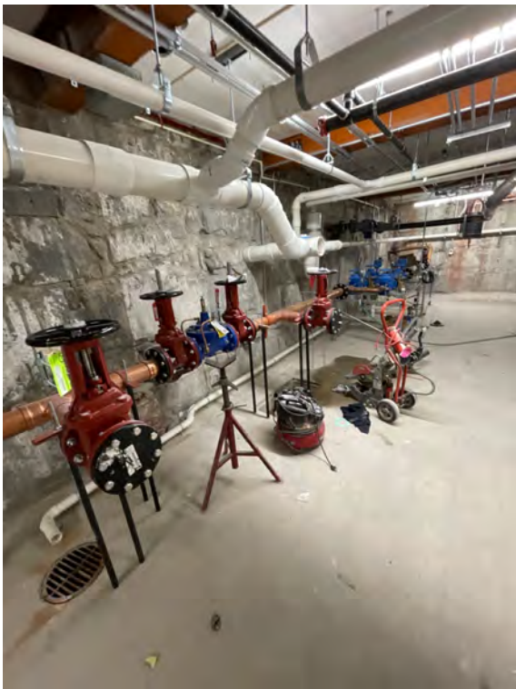
Description: Basement of existing building, domestic water service
