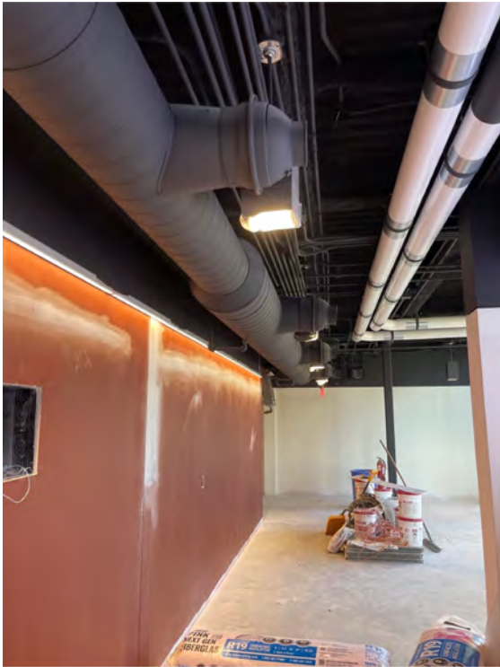
Description: Third-floor addition/spiral duct /registers grills and diffusers
