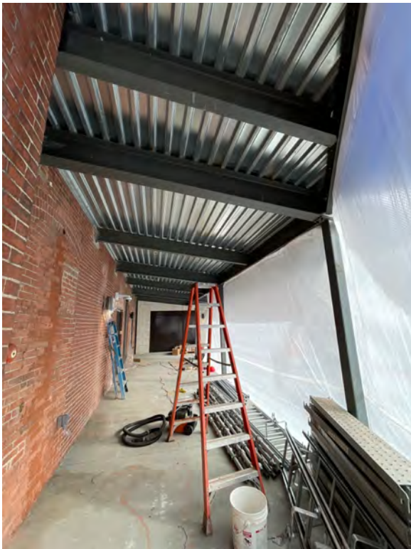
Description: Loading dock steel installed
