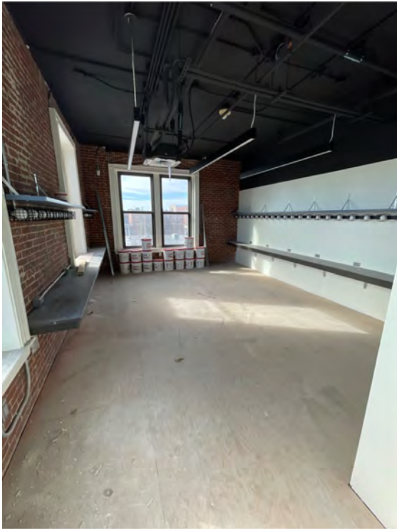
Description: Third-floor existing building dressing, room, millwork, and lighting installed
