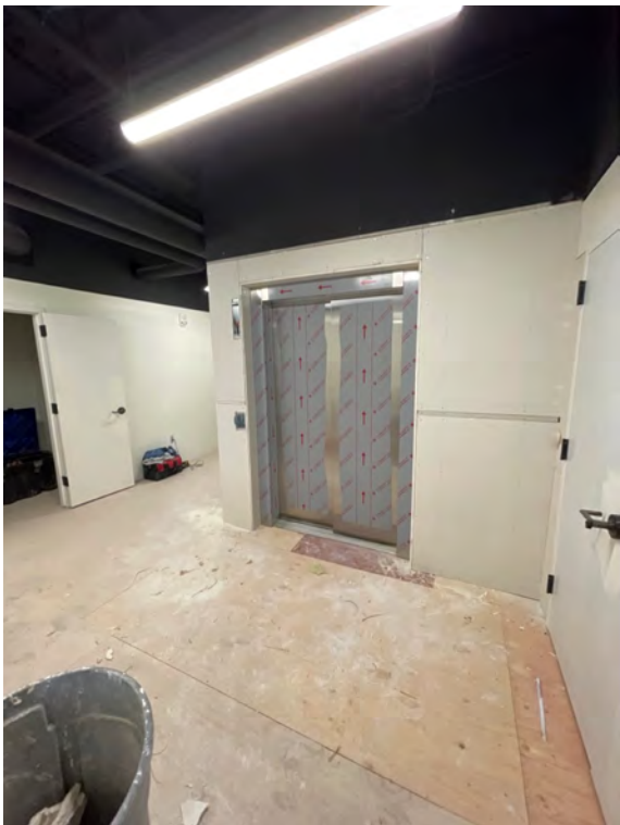
Description: Second floor existing building elevator installation
