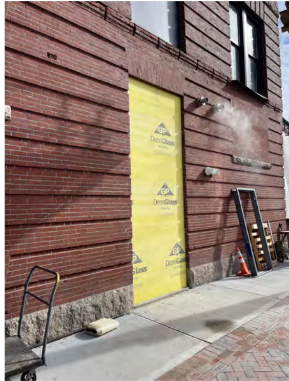
Description: Existing door infill at West elevation
